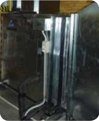
Image (B) Indoor Fan Coil Unit with EC Motor and Plug Fan.
