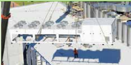
GEA Grasso ammonia chiller being installed on a building roof in Sydney
