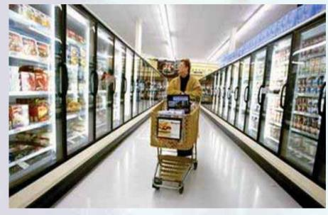
Doors on fridges do not stop people buying! In fact research shows that customers will spend longer in a refrigerated good section in areas fitted with doors as temperatures are not uncomfortable. Doors can save 30% to 70% of electricity use, savings equal to 20%+ return on capital not including depreciation
